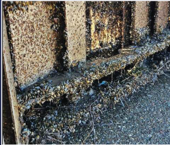
Gate covered by golden mussels (photo: DWR)
