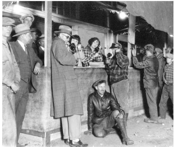
At an emergency telephone station, people seek information after the dam’s collapse.
