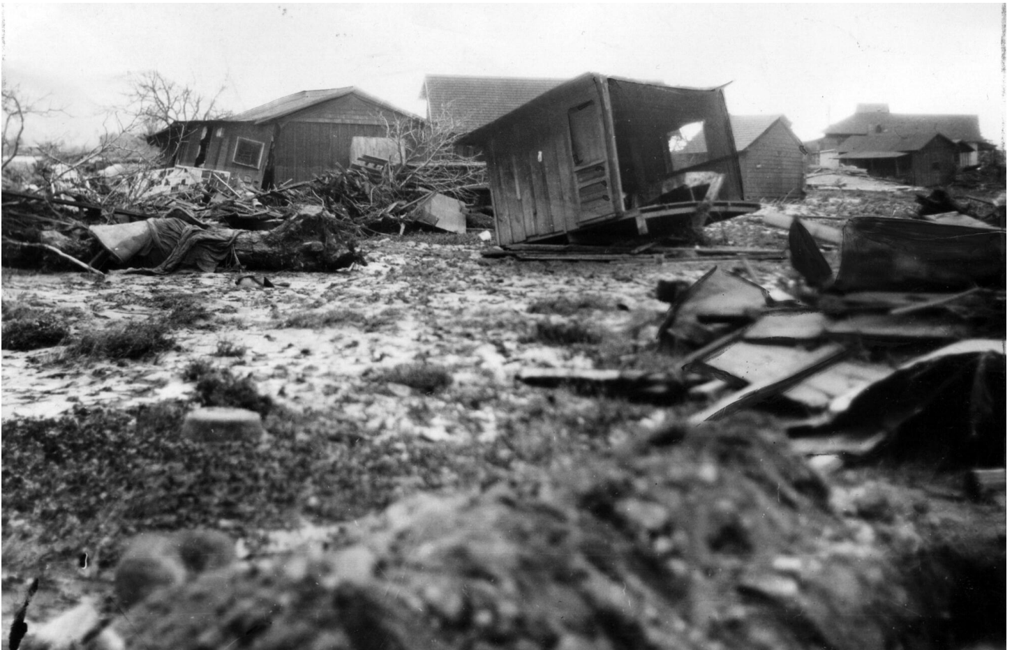
March 14, 1928: Remains of homes in Santa Paula following the collapse of St. Francis Dam.
