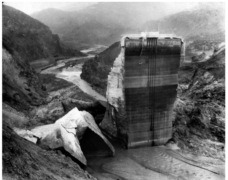
March 1928: The remaining section of the St. Francis Dam with crumbled sections at its base.
