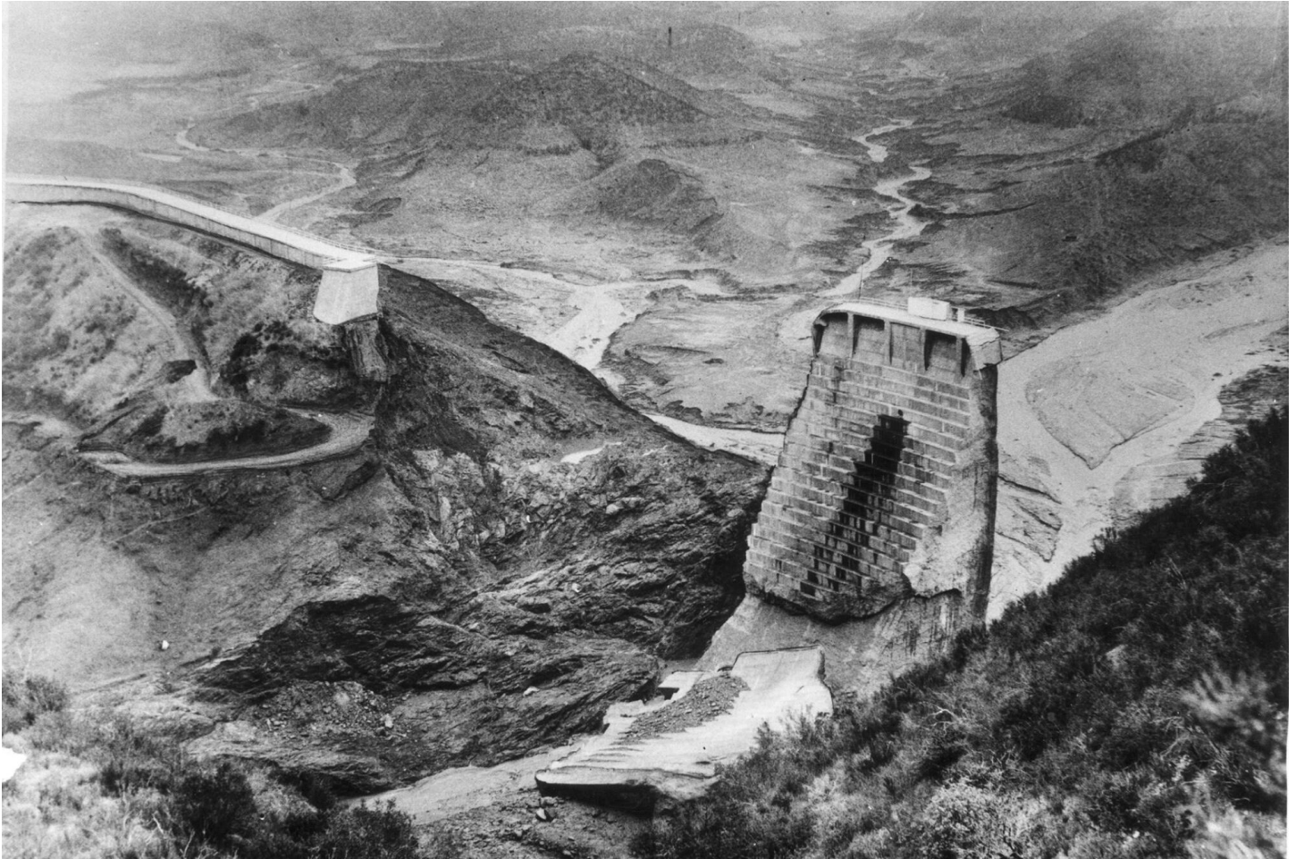
A 1928 photo of the St. Francis Dam after it collapsed and sent a 10-story wall of water through San Francisquito Canyon, killing more than 400 people.
