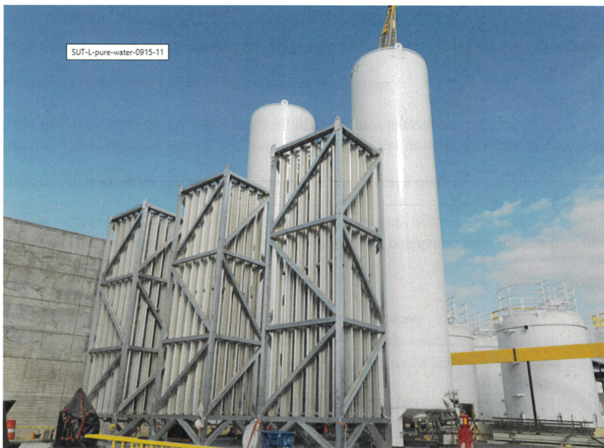
Liquid oxygen tanks at the Pure Water facility under construction in San Diego two years ago. (Ana Ramirez / The San Diego Union-Tribune)
